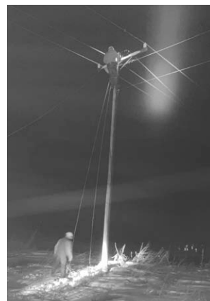
(right) A distribution pole is damaged by severe weather.
