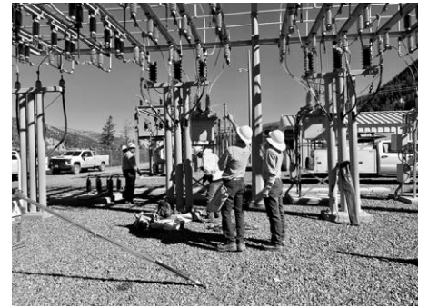
GCEA Linemen Discuss an outage in Lake City
