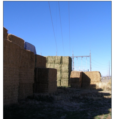
Stacking anything under power lines is risky. Equipment operators need to ensure they maintain the minimum 10-foot clearance from any power line with any part of their equipment or load.
