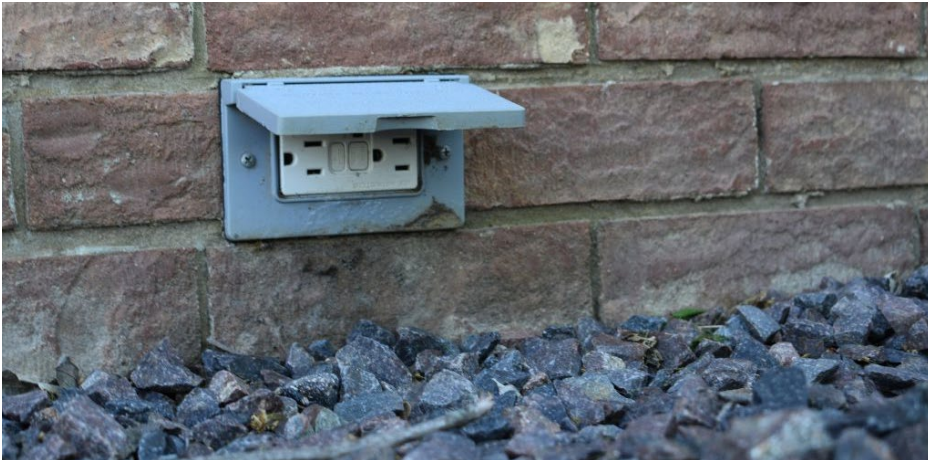
Use a GFCI outlet to power heat tape. Photo courtesy of SafeElectricity.org
