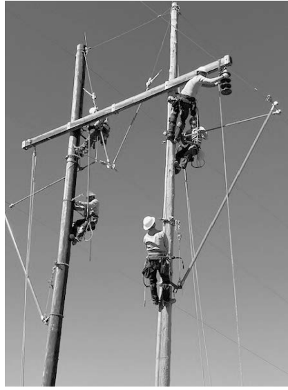
▲ A K.C. Electric Association construction crew replaces a crossarm on a 69,000-volt transmission H-Frame structure utilizing high-voltage hot sticks.
