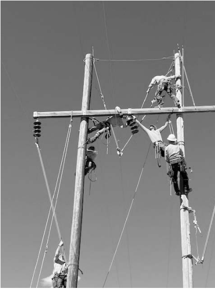
▲ A K.C. Electric Association construction crew replaces a crossarm on a 69,000-volt transmission H-Frame structure utilizing high-voltage hot sticks.
