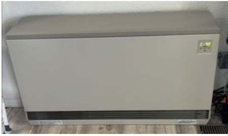
ETS heaters charge during times when electricity is in less demand and less expensive, storing heat in bricks and putting it right in the room where you want it, when you want it. Photo by Sabrina Shibe of Walsenburg.
