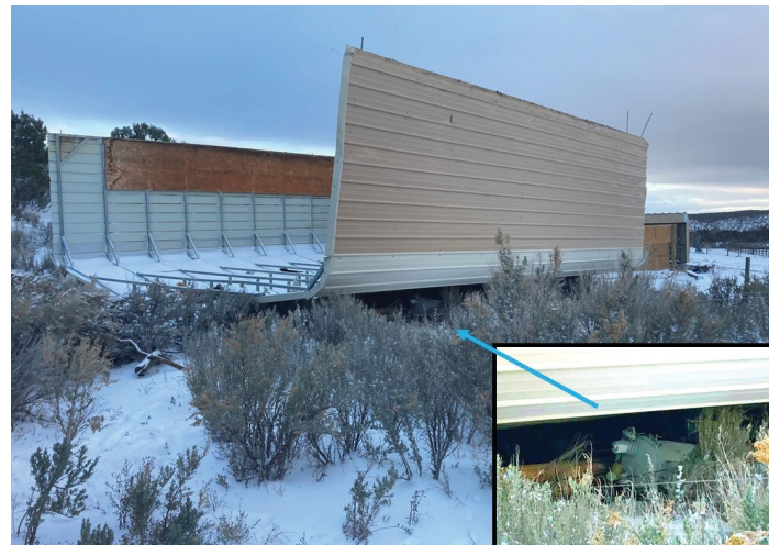
⬆ This carport was not properly anchored. During a spring storm, strong winds lifted the carport and dropped it on an EEA overhead line, breaking the pole and causing an outage for several members. Photo courtesy of Ken Tarr.
