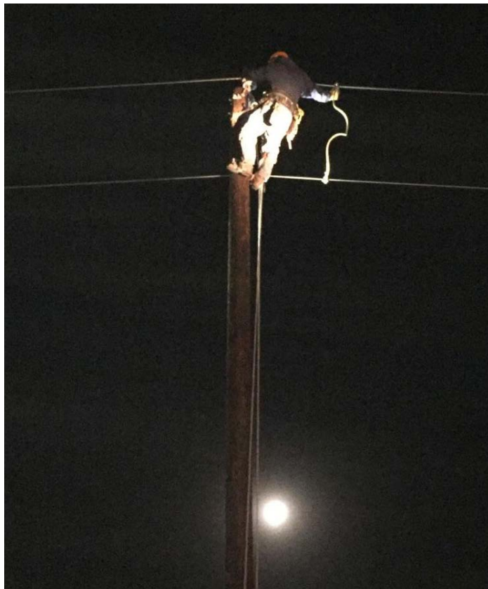
Shining under the full moon's glow, San Isabel Electric's dedicated lineworkers scale towering poles, alone, and in the dark, tirelessly restoring power to our communities.
