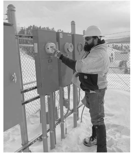
▲ Gunnison Lineman Justin Hulick removes a meter.
