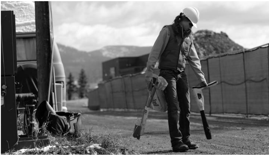
▲ Line Locator Lisa Lucas works to find and mark underground lines at a job site in Crested Butte..
