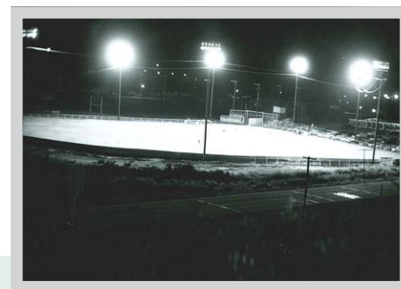
New ballfield lights installed in Craig
