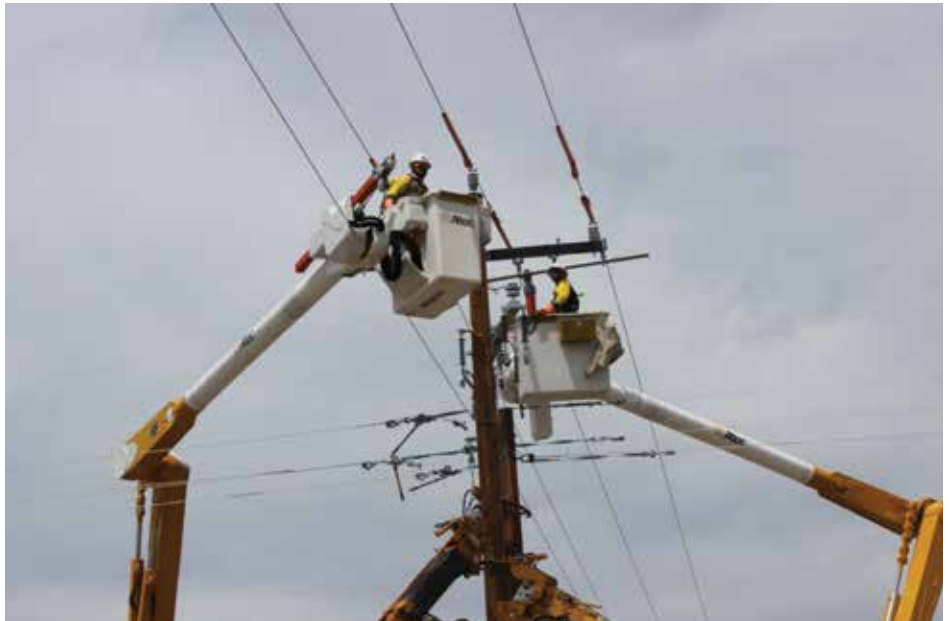
▲ EEA lineworkers perform hot line work with two bucket trucks.
