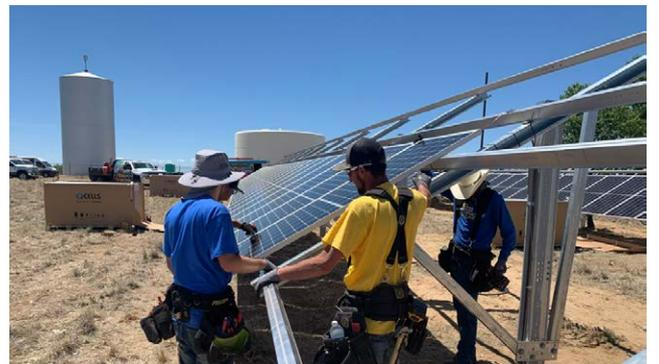
▲ **Steel City Solar technicians installed a 148 kilowatt solar array at the Newdale-Grand Valley Water Cooperative. The solar powered pumps help offset water distribution costs to residents and farmers in Otero County.**
