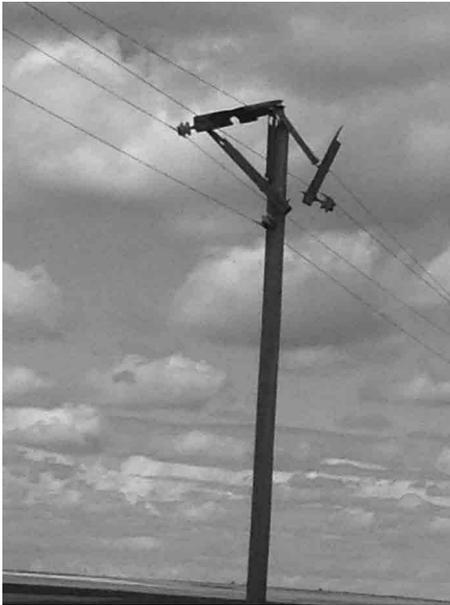
▲ This pole and cross-arm damage was caused by a wind storm.
