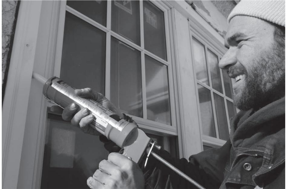
around windows, doors, electrical wiring and plumbing saves energy and money. There are many different types of caulking compounds available, but the most popular choice is silicone. Silicone caulk is waterproof and flexible and won't shrink or crack.
